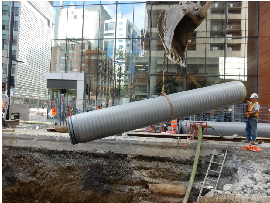
Figure 4.5: Triple wall corrugated pipe installation
