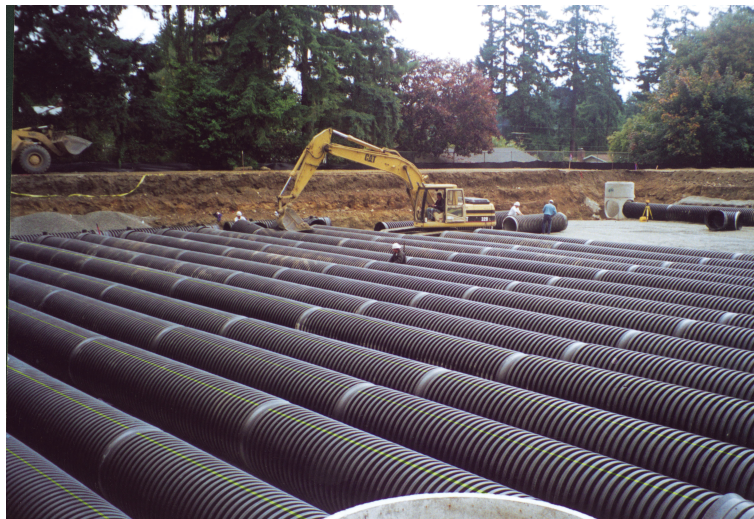
Figure 4.11: Typical detention system
