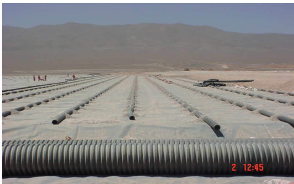
Figure 4.14: Typical heap leach pad construction
