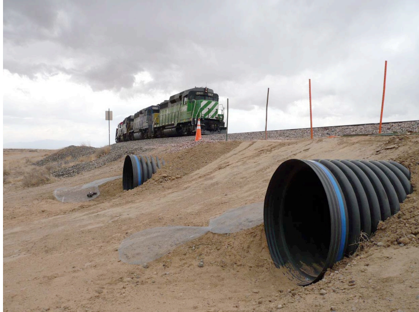
Figure 4.9: AAR TPCI test installation in progress
